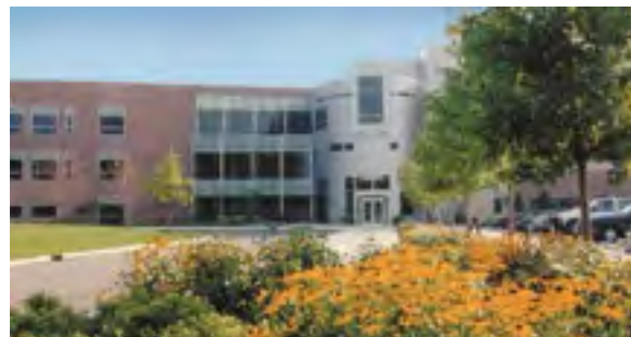
Parker Hannifin Corporation Headquarters Cleveland, Ohio
