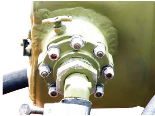
Figure 9-3. Oil Tank sump and drain valve.
